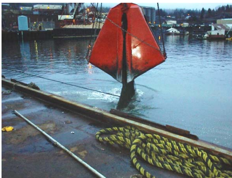
Figure 3. Thin-layer placement in Ward Cove.
